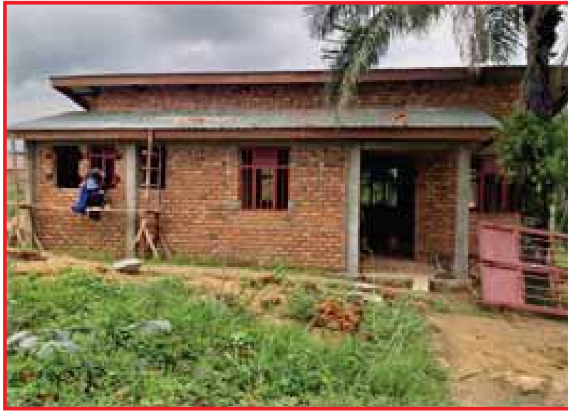
Photo 10 : Tshikapa skills Lab under construction
